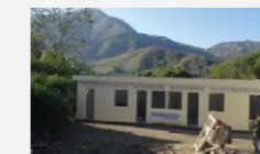
Restroom and water supply facilities upon completion © Plan International Japan
